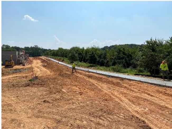
Figure 5: Site perimeter sidewalk installation underway
