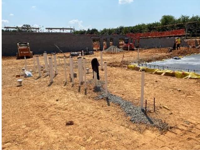
Figure 2: Upper slab plumbing is backfilled and compacted.
