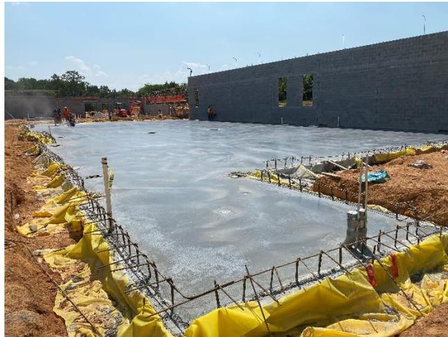
Figure 1: Depressed Slab Installation
