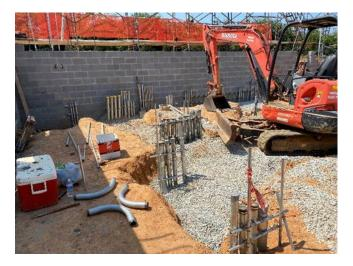
Figure 3: Electrical room conduit & slab prep underway
