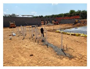
Figure 2: Upper slab plumbing is backfilled and compacted.
