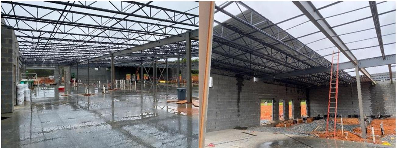
Figure 1: All lower and upper roof structure is set, roof decking underway
