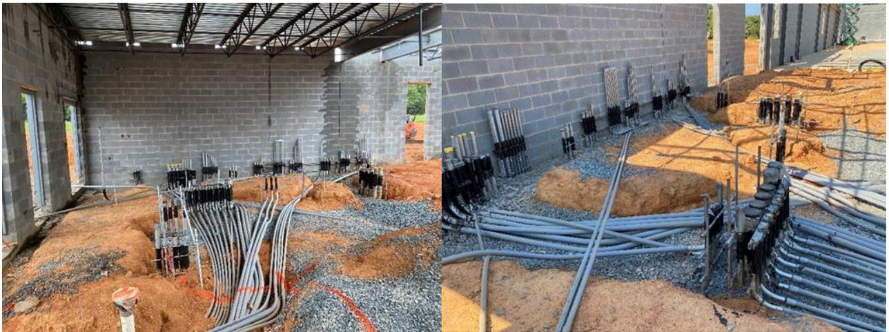
Figure 3: Electrical / data center room conduit work continues
