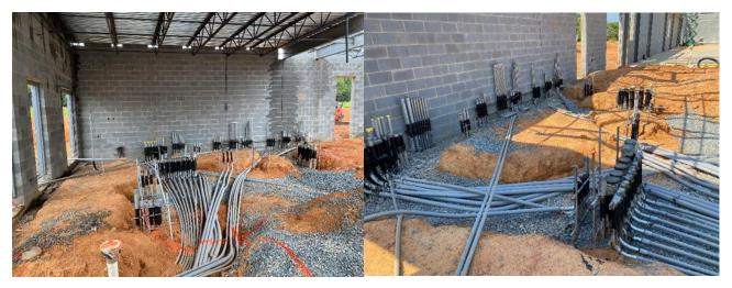
Figure 3: Electrical / data center room conduit work continues
