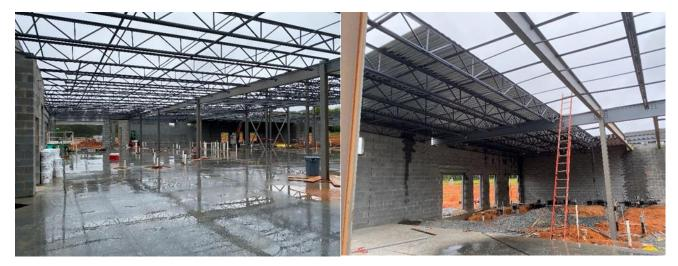
Figure 1: All lower and upper roof structure is set, roof decking underway
