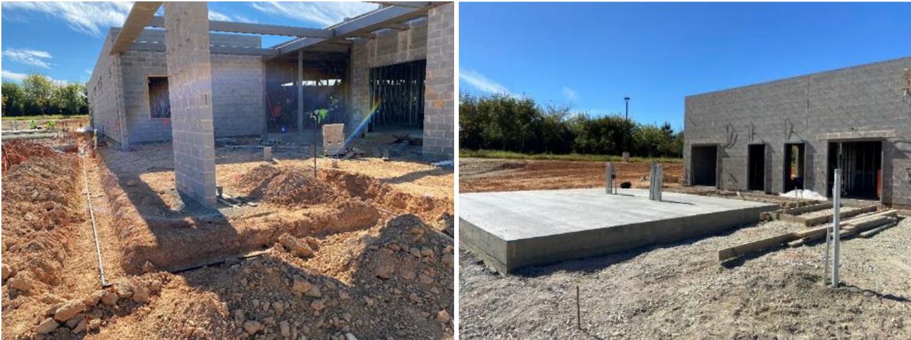
Figure 3: Exterior utility provisioning in process
