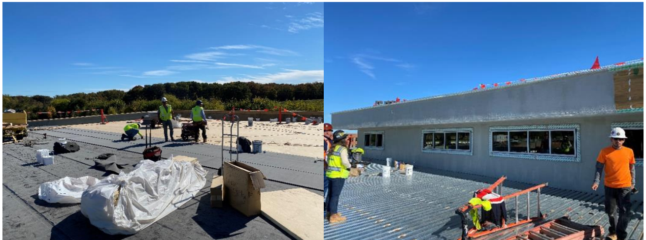
Figure 1: Installation of roofing and upper exterior windows underway
