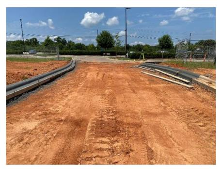
Figure 4: Curb and gutter for parking/driveways underway
