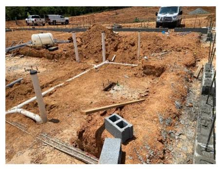
Figure 2: Under slab rough-ins underway
