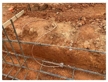
Figure 5: Grounding installation in progress
