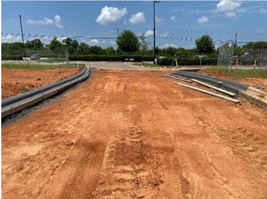
Figure 4: Curb and gutter for parking/driveways underway
