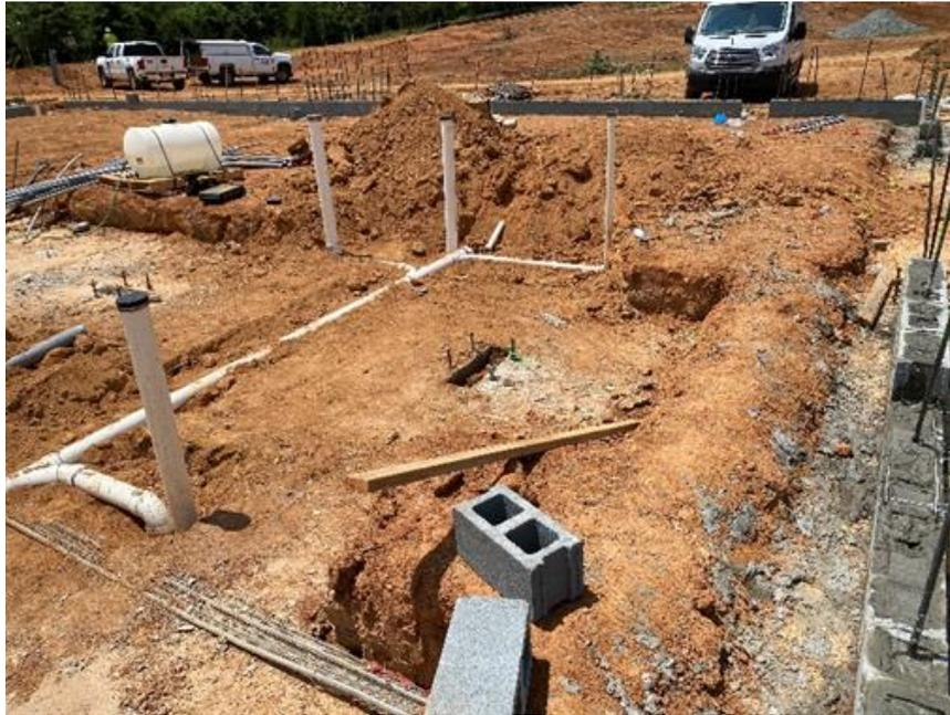
Figure 2: Under slab rough-ins underway
