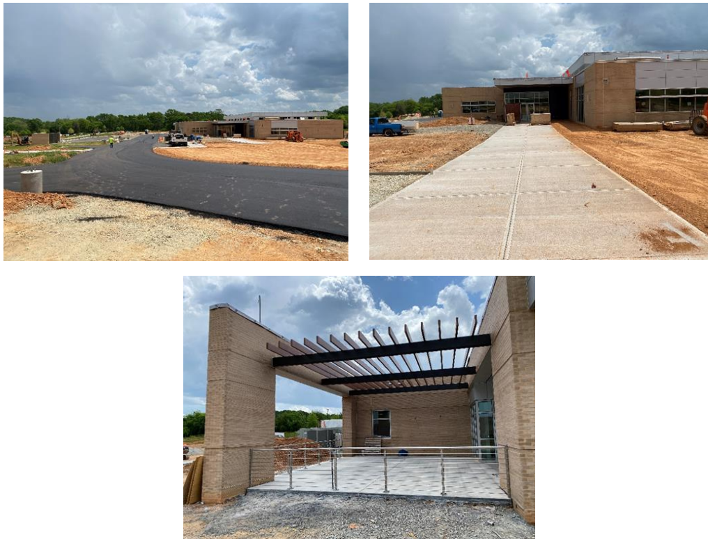
Figure 3: Building exterior, site paving and concrete installation underway
