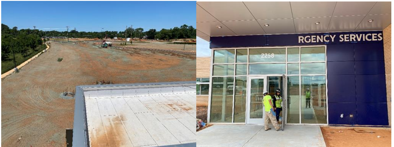
Figure 3: Site finish grading completed and seeded; Building exterior finishes in progress
