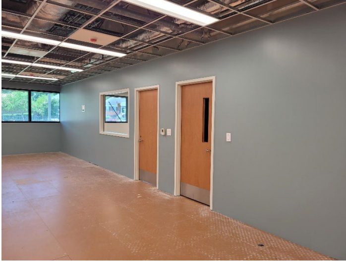
Internal doors installed
