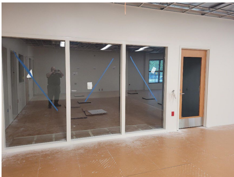
Internal glass installed.
