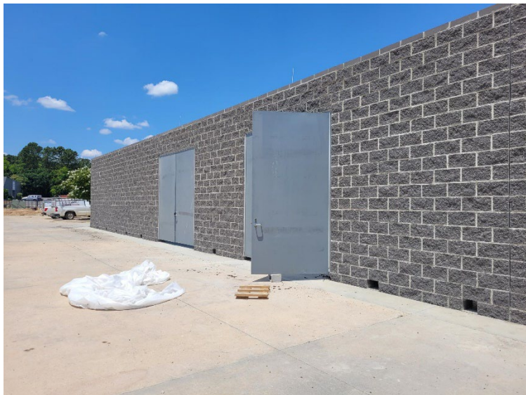
Doors for Mechanical yard installed
