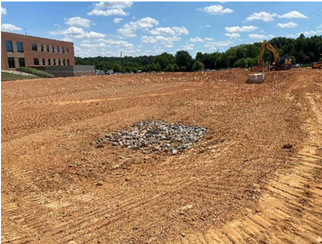
BMP 95% built, rip rap starting, then seeding
