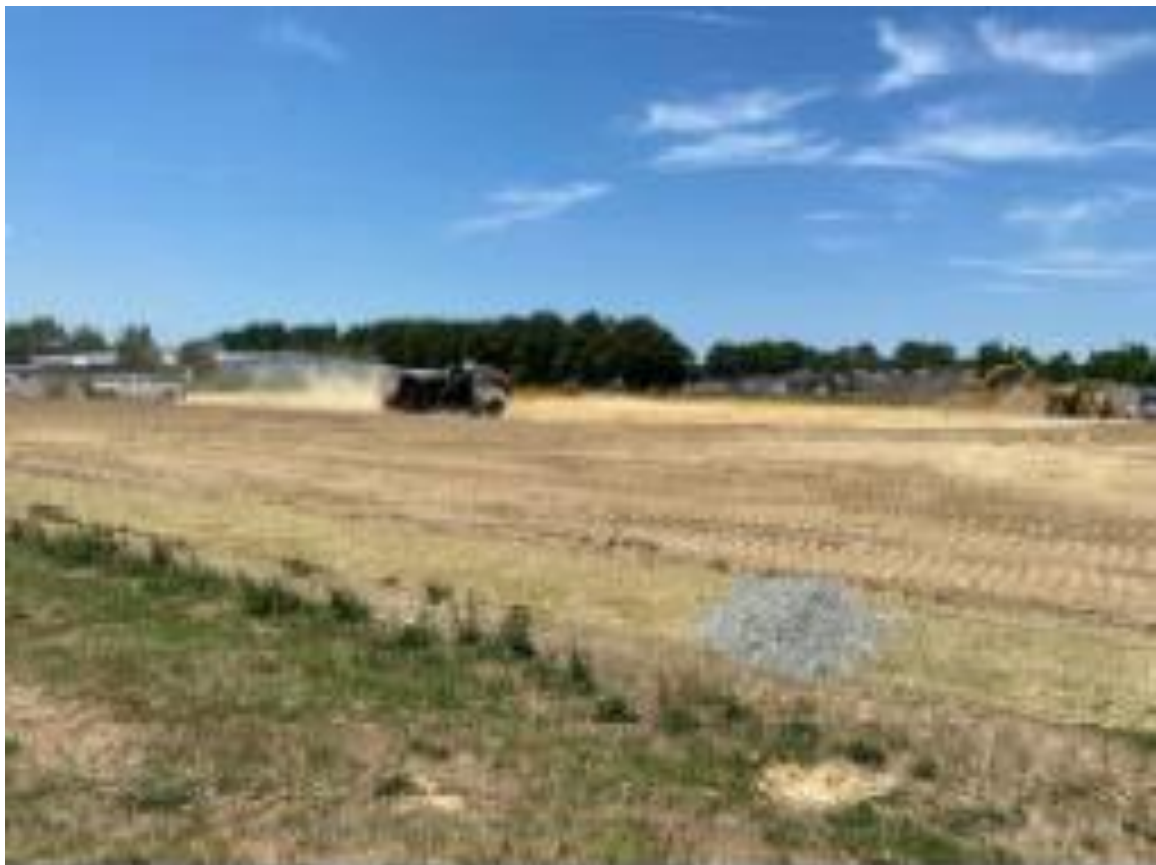
Figure 1: Structural Fill Delivery
