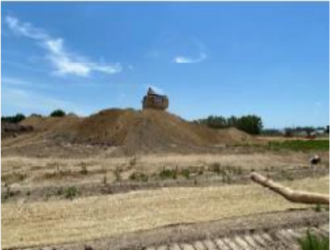
Figure 2: Stockpile Structural Fill
