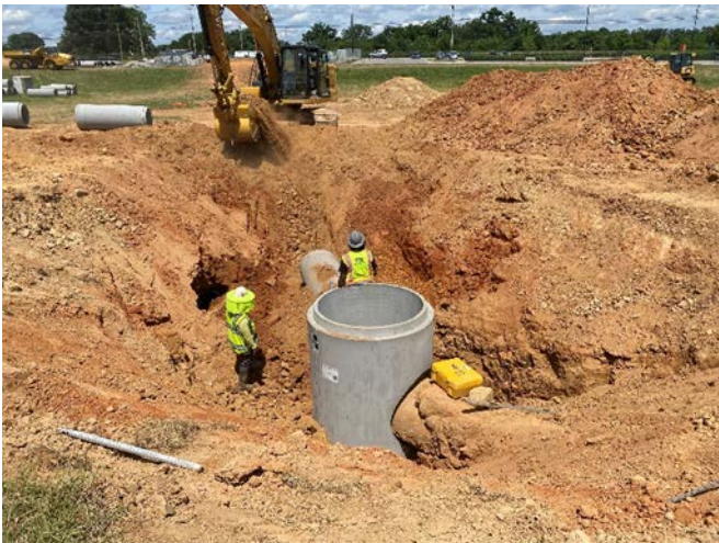
Existing site storm water system relocation underway
