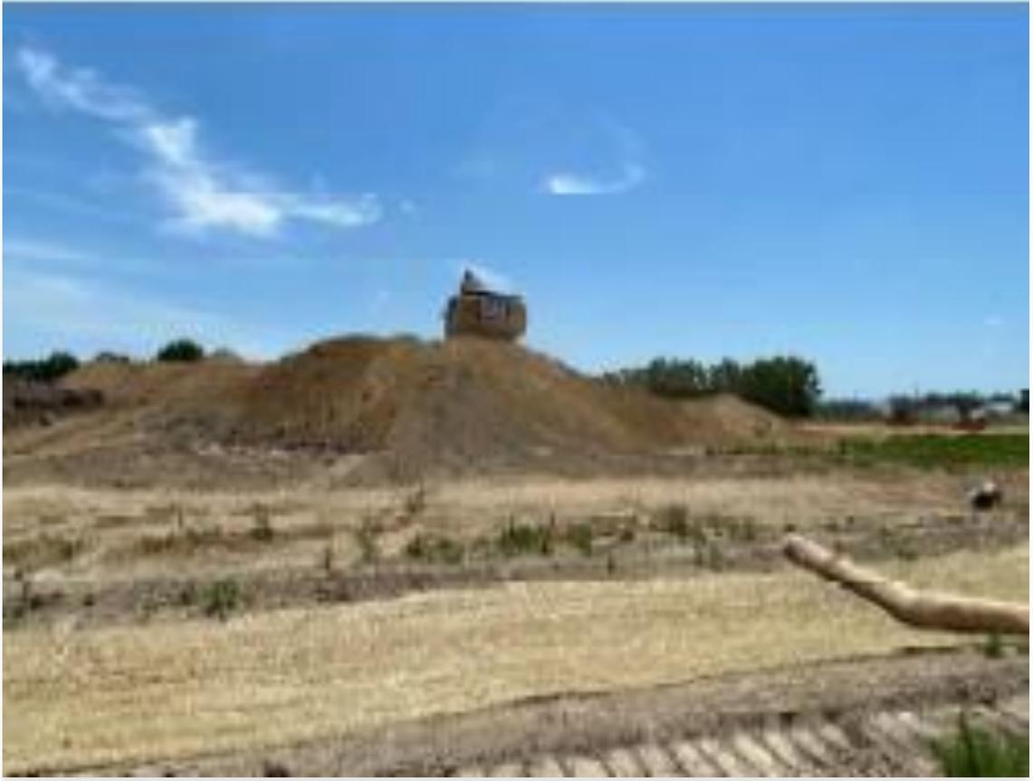
Figure 2: Stockpile Structural Fill
