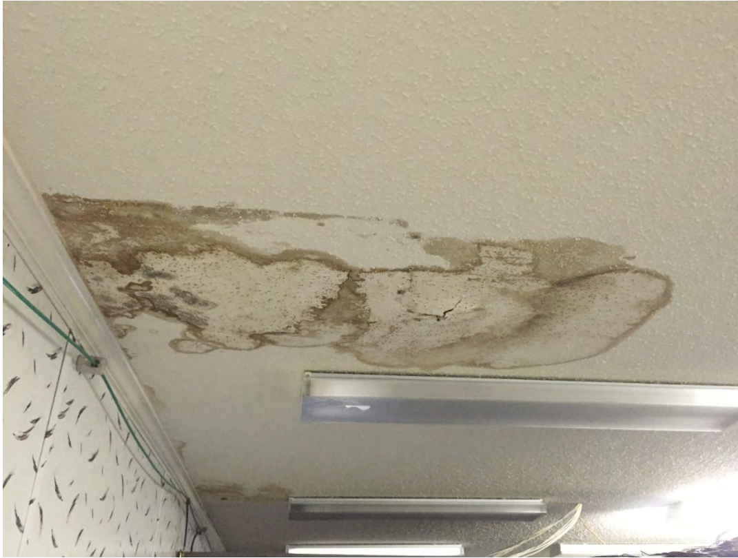
Figure 11 – Roof Leak
