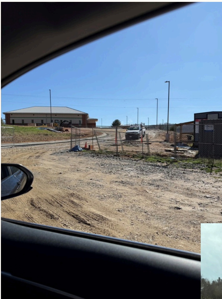
Yancey County's New 911 Center
