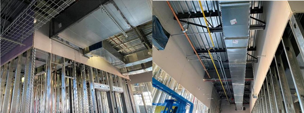
Figure 2: Interior wall framing completed; Gas, water, fire alarm, power & ducts in progress.
