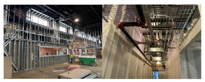
Figure 2: Rough ins and wall completions for 911 & EOC areas in progress. Supporting infrastructure for structured/low voltage cabling and other systems underway.
