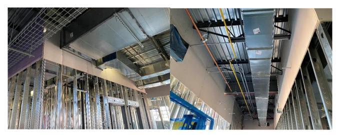
Figure 2: Interior wall framing completed; Gas, water, fire alarm, power & ducts in progress.
