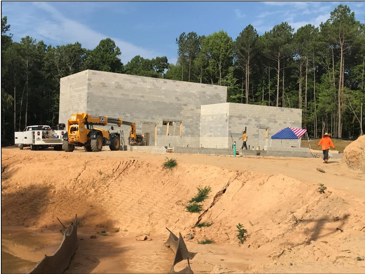
Figure 1: Load Bearing Masonry Underway (7/27/2022)
