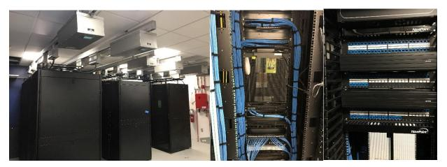
Figure 1: Data center equipment racks installed, and structured cabling terminated
