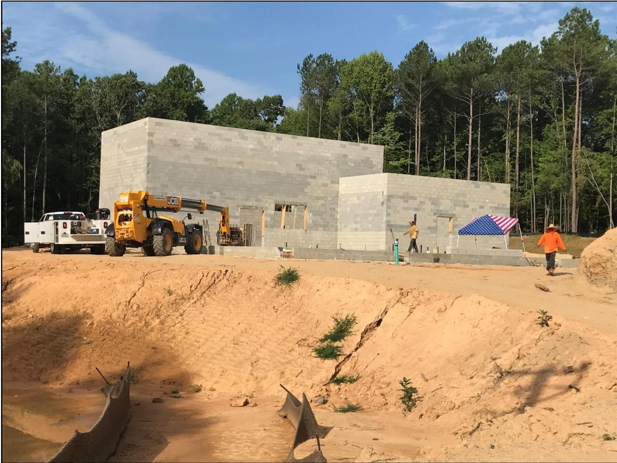
Figure 1: Load Bearing Masonry Underway (7/27/2022)
