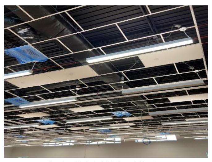
Figure 3: Suspended ceiling installation in all areas of building underway
