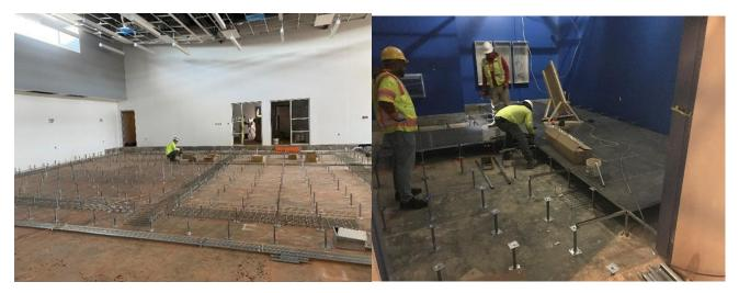
Figure 1: Conduit, wiring trays and access floor installation in progress
