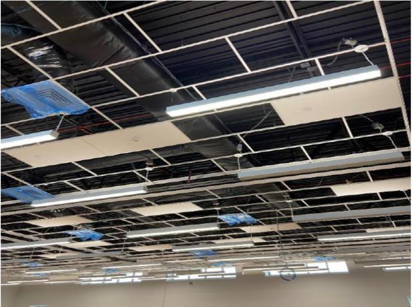
Figure 3: Suspended ceiling installation in all areas of building underway
