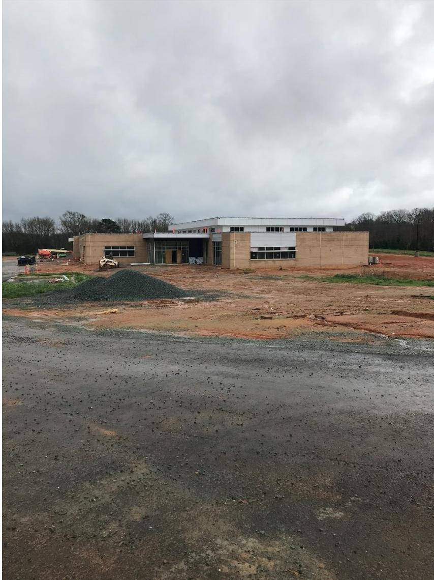
Figure 2: Finish grade around building starting
