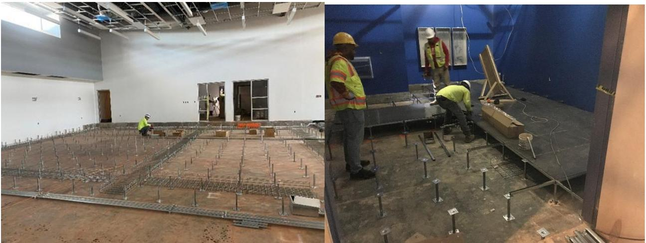
Figure 1: Conduit, wiring trays and access floor installation in progress
