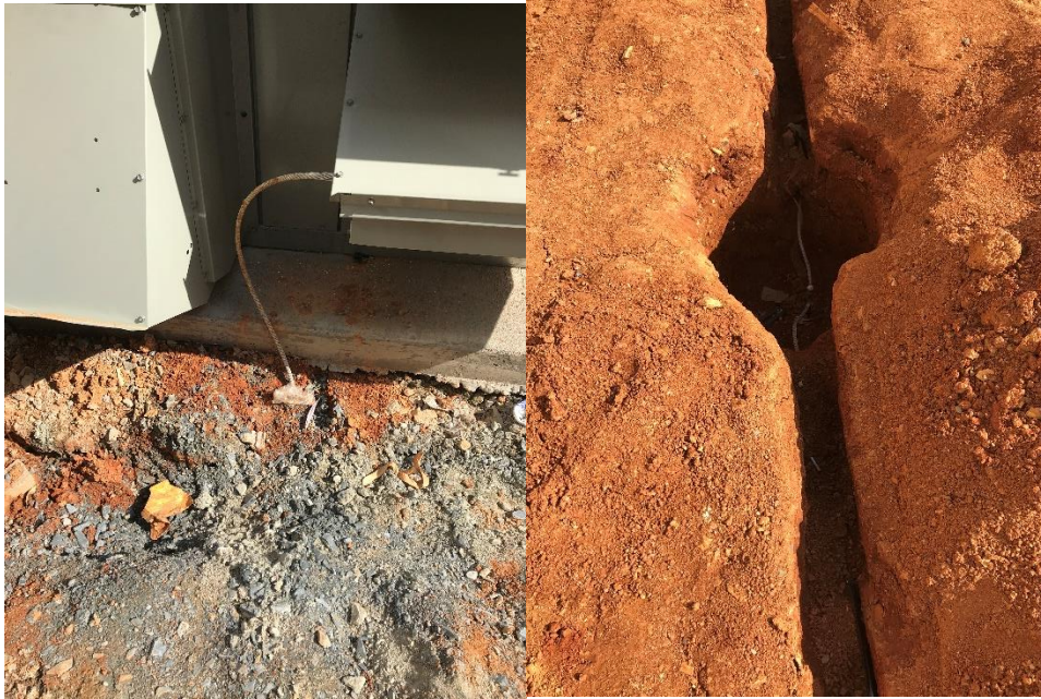
Figure 2: Exterior ground ring installation
