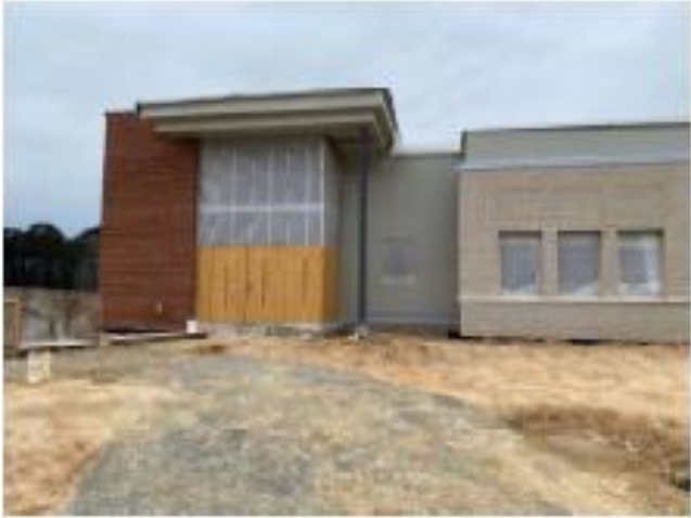
Condition at Staff Entry
