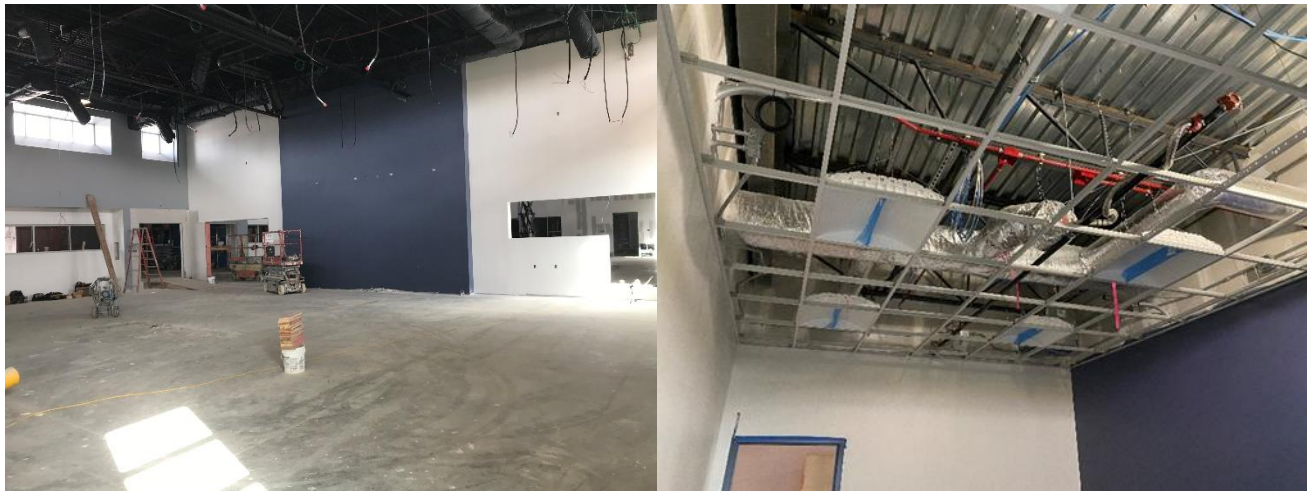
Figure 1: Interior painting , tile & ceiling grid work
