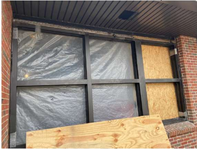
New Store front installation.
