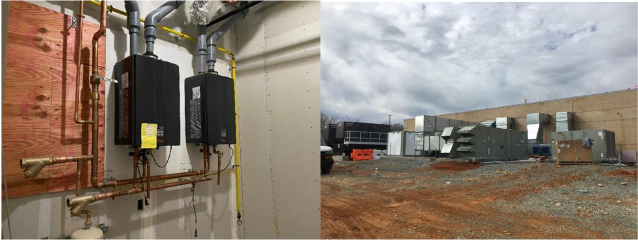
Figure 3: Plumbing and mechanical systems installations continue.
