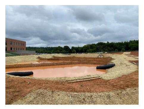
Figure 1: BMP completed & functional
