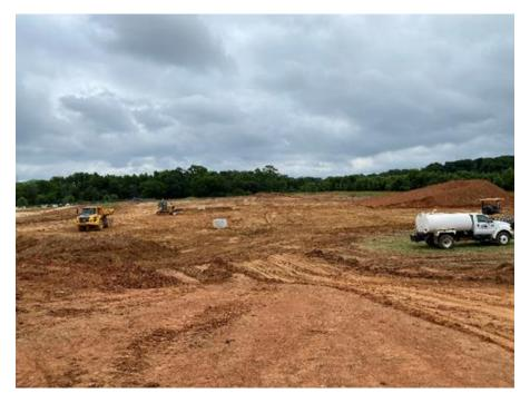
Figure 2: Additional site grading underway
